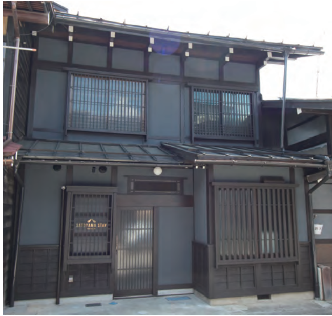
Entrance is at west side of the building.
